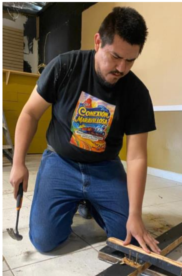
Christian doing construction on the church building
